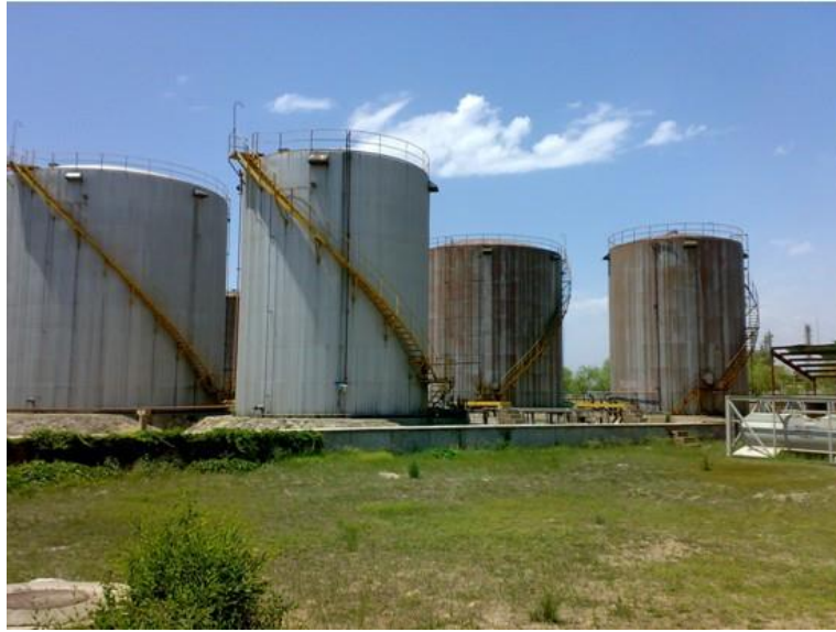
Appearance of atmospheric tank to be tested
